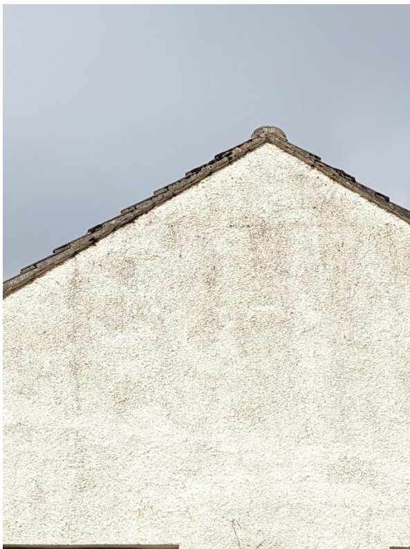
Photo 15 – Cracking to wet verge to left elevation
