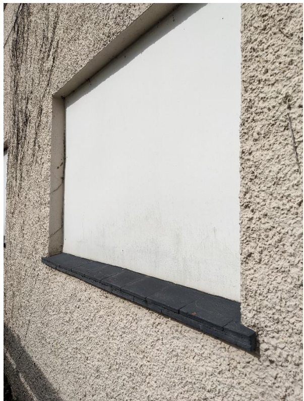
Photo 16 – Blocked up window to left elevation and tiled windowsill
