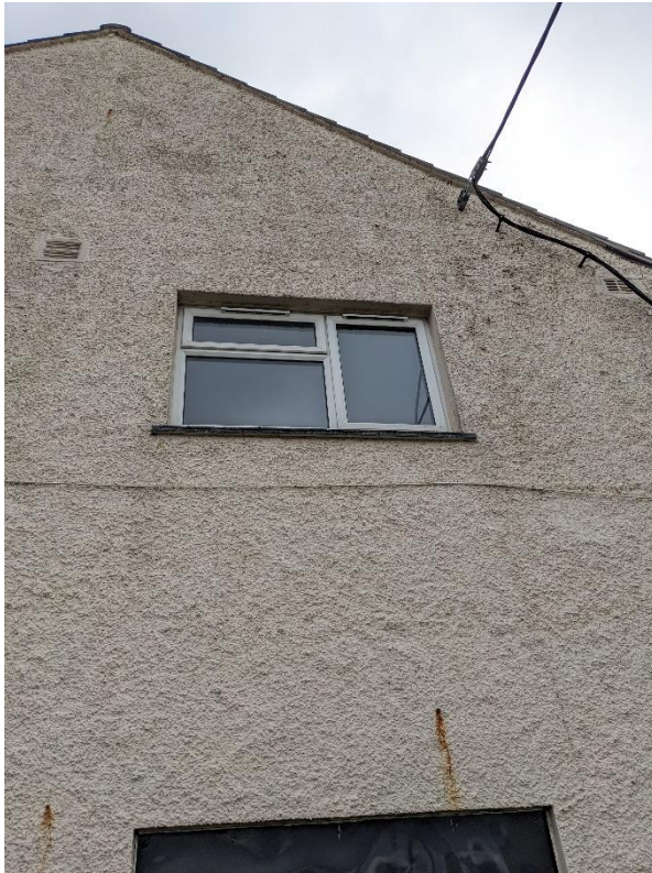
Photo 21 – Cracking below window to right elevation
