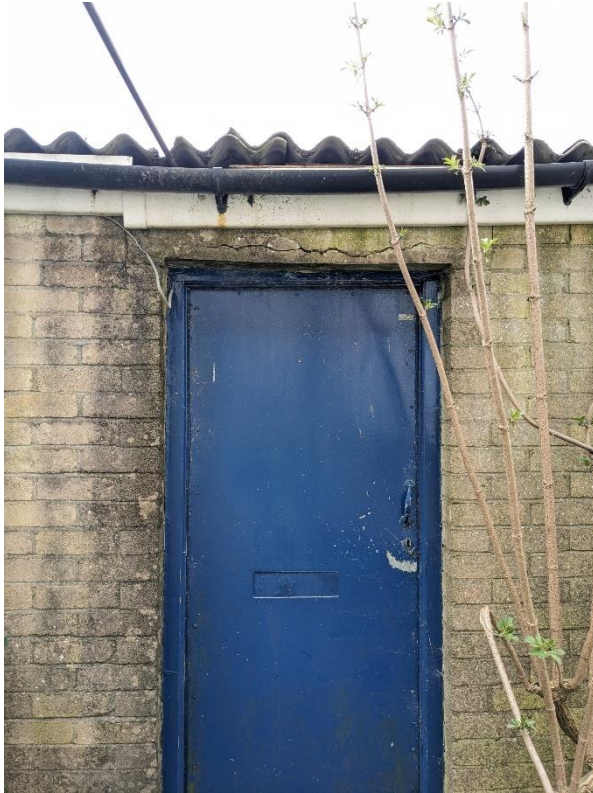
Photo 25 – Cracked lintel above front door of outbuilding
