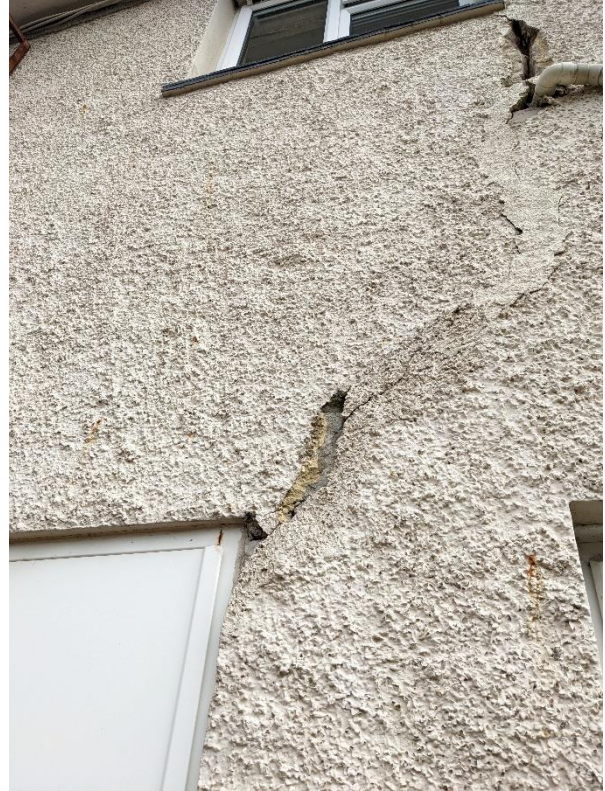
Photo 18 – Blown render around cracking to rear elevation
