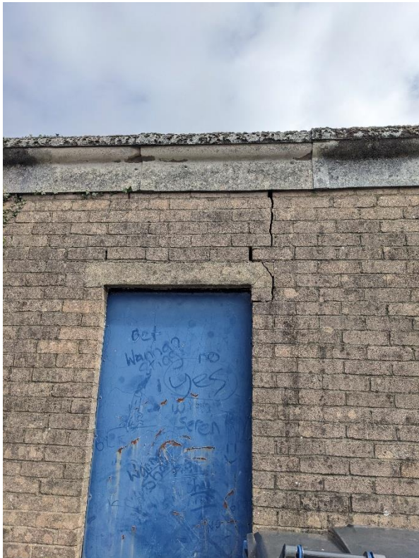
Photo 27 – Cracking to rear of outbuilding
