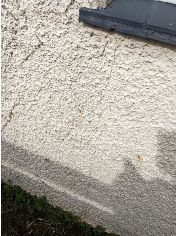
Photo 17 – Cracking below window to left elevation
